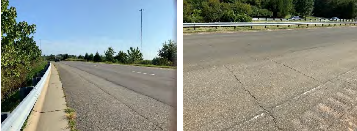
Figure 3: Pavement Striping Inspection Results Sample
