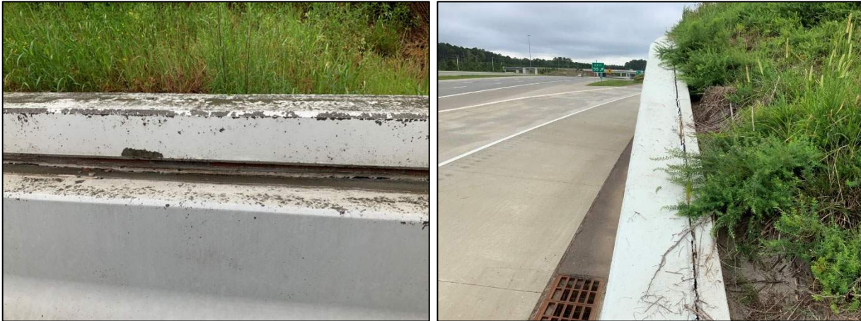
Figure 3: Retaining and Sound Barrier Walls Inspection Results Sample
