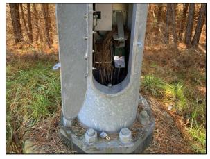
To increase future highway lighting ratings, it is recommended that all damaged highway lights noted during the inspection be repaired and/or replaced in accordance with the *NCTA Roadway and Facility Maintenance Standards V6*, referenced below. Additional care should be taken to ensure all access panels are properly secured to prevent rodent and other animal intrusion.
