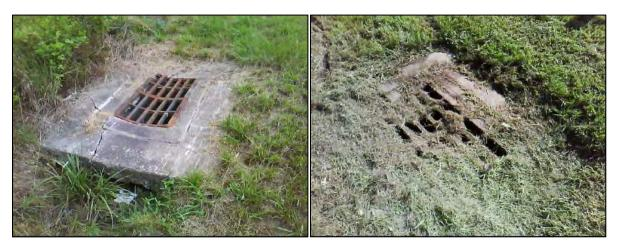
To improve inlet performance throughout the facility, it is recommended that the maintenance provider inspect inlets pursuant to the *NCTA Roadway and Facility Maintenance Standards V4*, referenced below. During inspections, it is also recommended that the maintenance provider remove any debris accumulation upon observation.
