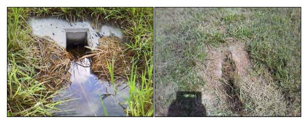
**Figure 4: Miscellaneous Drainage Failures**
