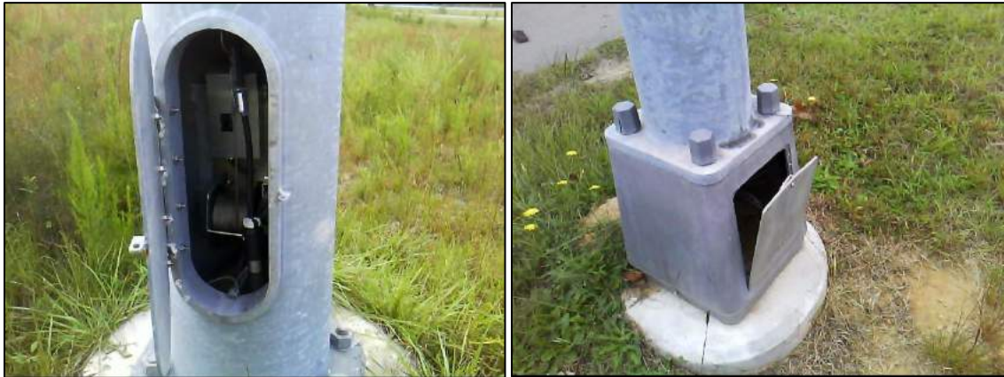
Figure 7: Highway Lighting Inspection Results Sample
