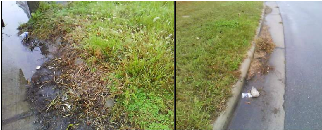
Figure 3: Curb and Gutter Inspection Results Sample
