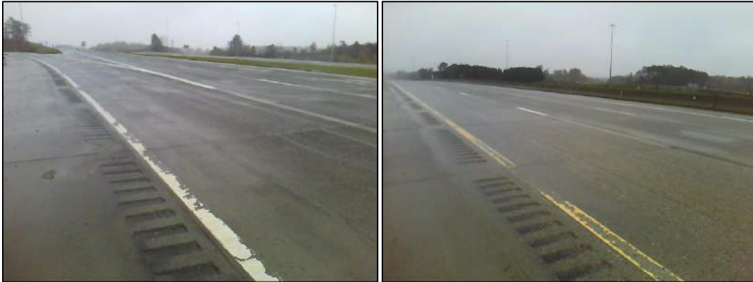
Figure 6: Pavement Striping/Marking Inspection Results Sample
