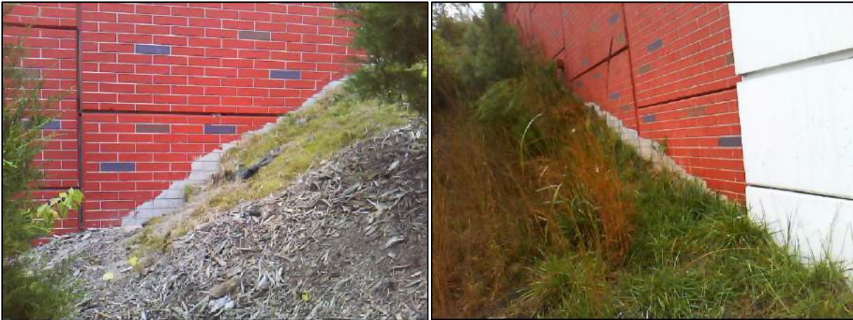
Figure 5: Retaining and Sound Barrier Walls Inspection Results Sample
